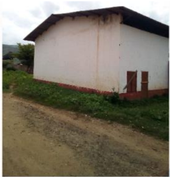
Village Mananasy -Maison de stockage
